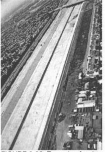
FIGURE 3-25 Example of a channelized urban stream for maximized flood conveyance and geomorphic stability (Los Angeles River, California). SOURCE: Reprinted, with permission, from Water Resources Research. Copyright by the American Geophysical Union.
