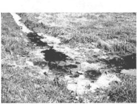
Failing sanitary sewer, causing upwelling of sewage through soil, and draining to gutter and then to storm drainage system. SOURCE: Robert Pitt.
